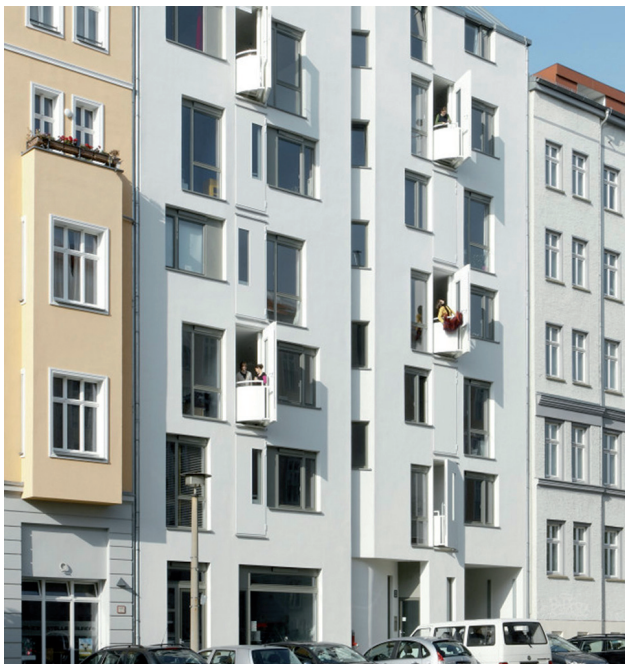
Fig. 9. Strelitzer Strasse Berlin, co-housing project 13
