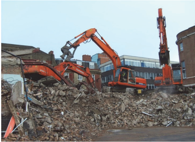
Fig. 1.2. The beginning of demolition waste processing (photo by J. Katzer)
