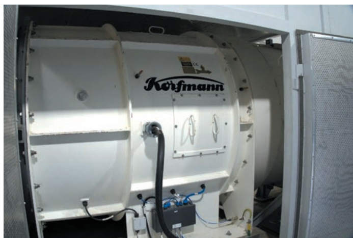
Fig. 4. Fan type dAL16-1100 manufactured by Korfmann
