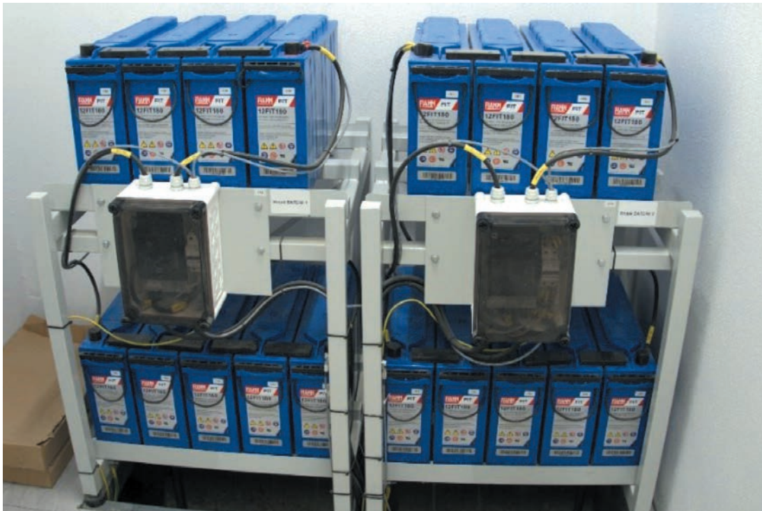
Fig. 8. Accumulator batteries
