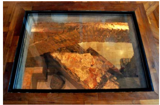
Fig. 9. A "window" in a floor with a view of basement. Source: K. Wierzbicki, February 2017
