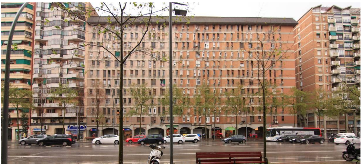
Fig. 8. MBM. Housing building in carrer Pallars. Source: Photo by M. Lucchini
