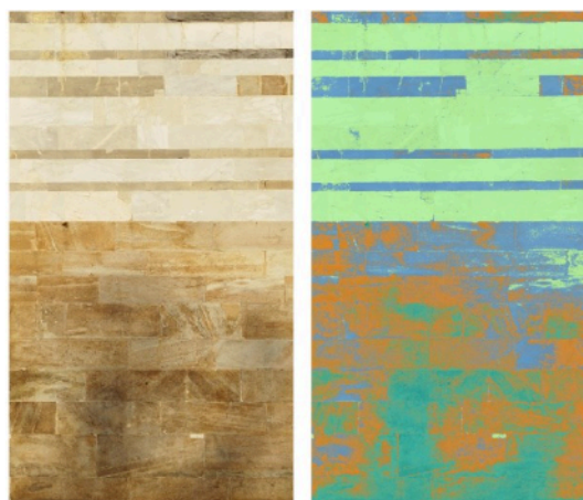
Fig. 7. The SOM clustering results (on the right) compared to the original ROI (on the left). Green = Segment 1; brown = Segment 2; blue = Segment 3; cyan = Segment 4.
