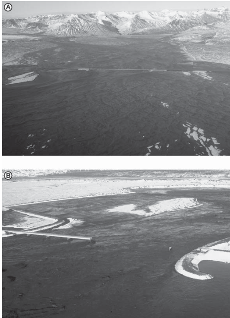
Fig. 2. The destructive power of the 1996 Vatnajökull jökulhlaup. A: On 5 November 1996 at 14.40 h. The 900 m long Skeiðará bridge and protective dike system over the river are still intact, in spite of the high discharge of 15,000 \text{ m}^3 \text{ s}^{-1} . B: The discharge (about 5,000 \text{ m}^3 \text{ s}^{-1} at this time, a few hours after the situation shown in Figure 2-A) has diminished, but the eastern end of the bridge crossing the streamway over the sandur plain has been washed away in the meantime.
