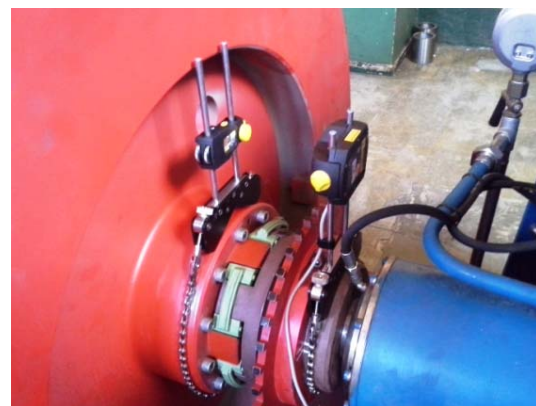
Fig. 7. Laser encoder with reflector used during shaft alignment.
