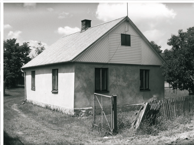
Fig. 2/a-d. Rammed earthen farmhouses in Tworkowice; source: the authors, 2009
