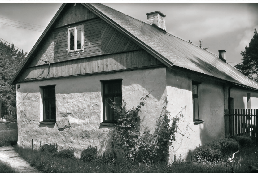
Fig. 2/a-d. Rammed earthen farmhouses in Tworkowice; source: the authors, 2009
