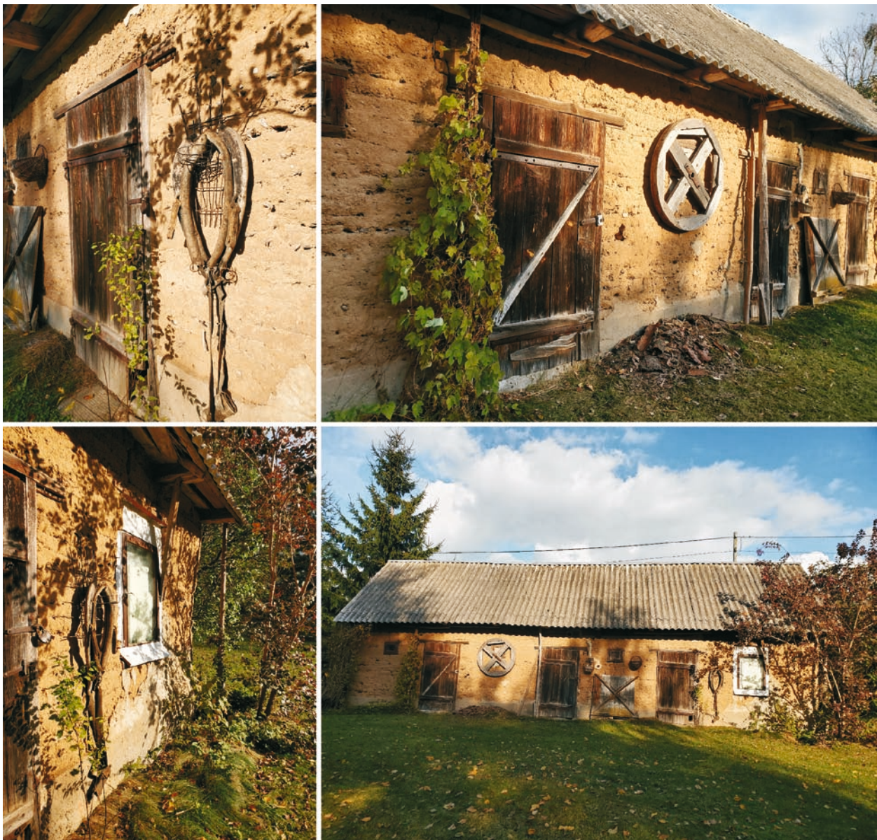
Fig. 9/a-d. A rammed earthen barn in Tworkowice; source: the authors, 2021
