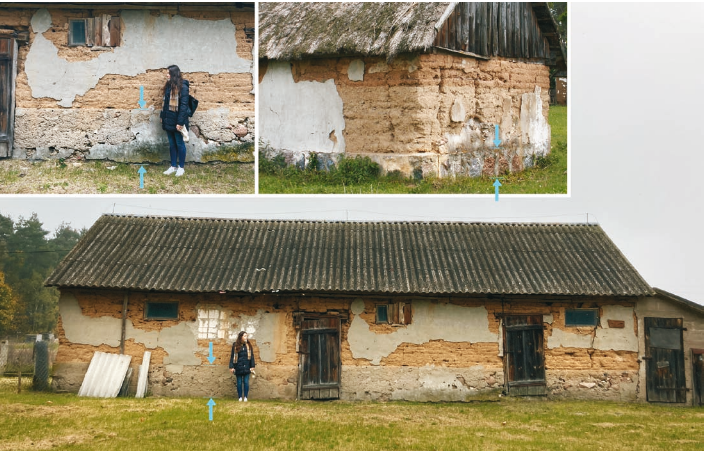
Fig. 10/a-c. Elevated foundations of rammed earthen barns; source: the authors, 2021
