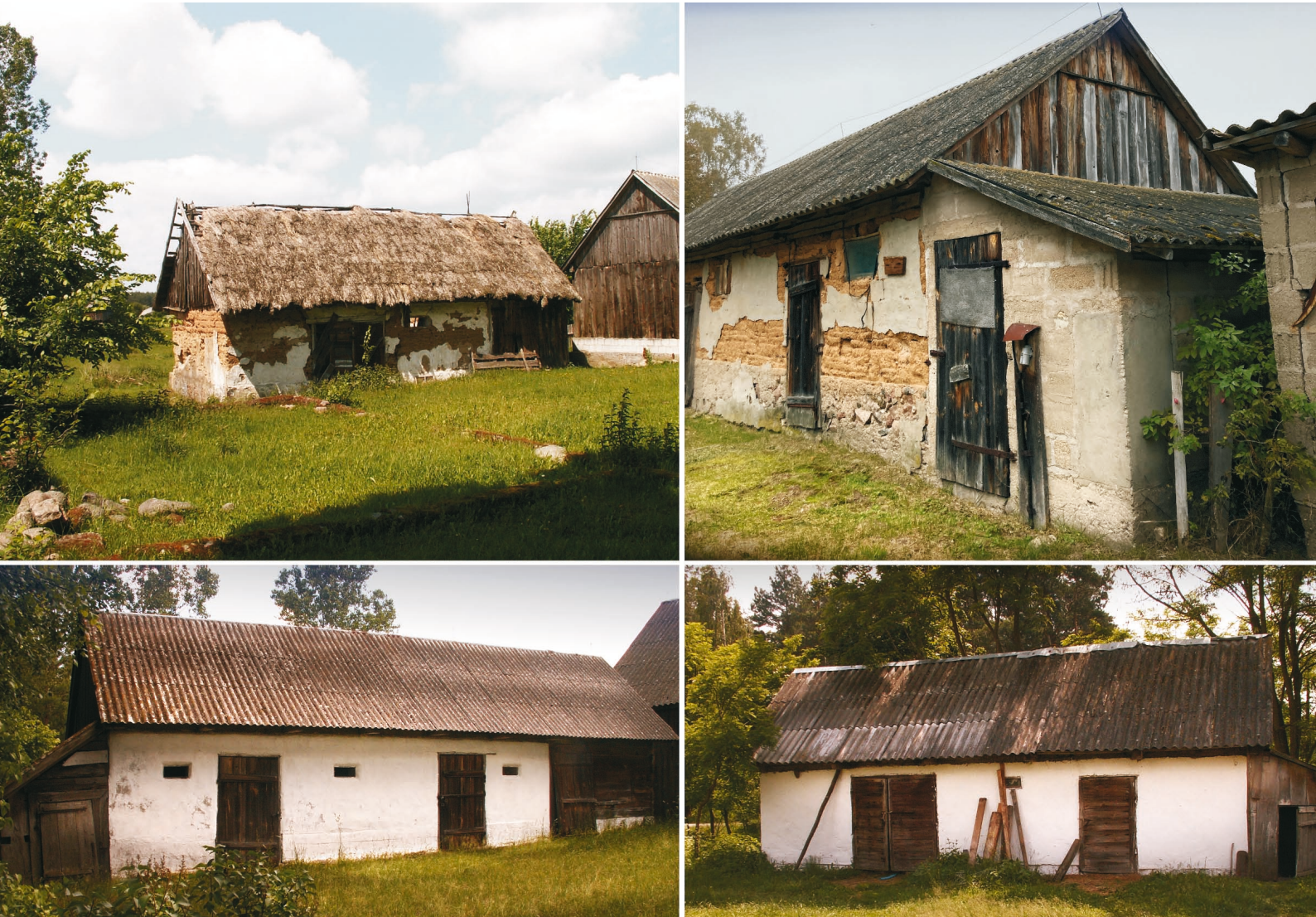
Fig. 8/a-d. Rammed earthen barns in Tworkowice; source: the authors, 2009 (a, c, d) and 2021 (b)
