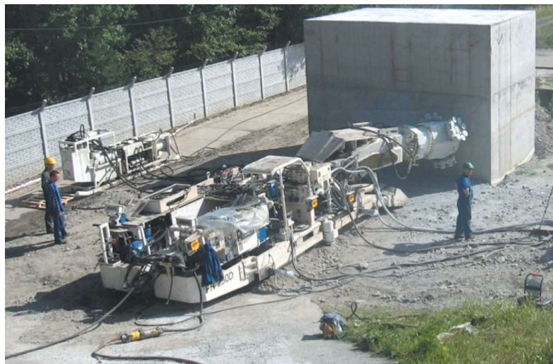
Fig. 8. View of mining head with disc tools mounted on type FR 250 roadheader during field tests
