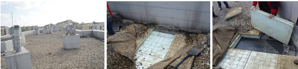
Fig. 1. View of the tested roofs
