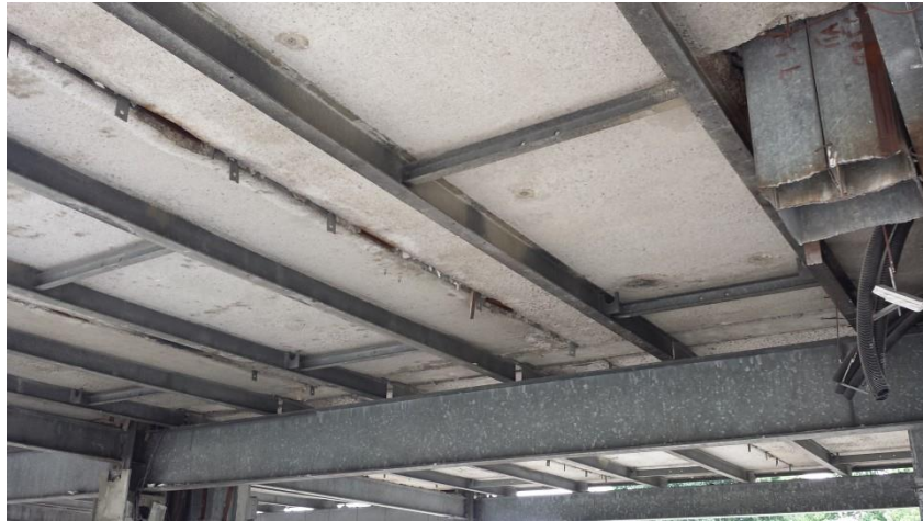
Fig. 6. View of prefabricated building modules of Lipsk type building
