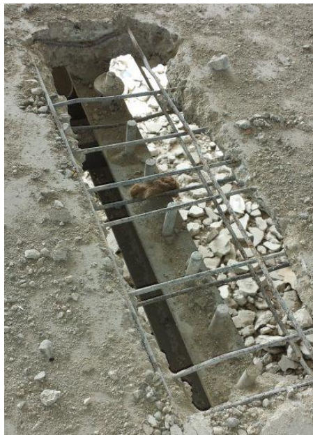
Fig. 7. View of fasteners and reinforcement bars
