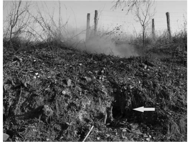
Fig. 3. Using smoke bombs to detect connectivity of soil pipes. A pipe outlet is in the foreground, smoke is rising from the opening sinkhole on the slope in the background
