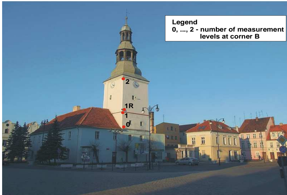
Fig. 3. Measurement levels on brick section of the tower
