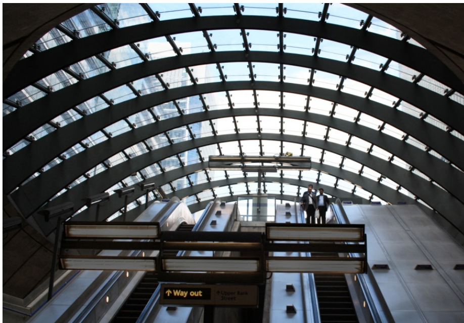
Fig. 5. The glass roof covering the entrance to the metro station Canary Wharf , London (Photo: Katarzyna Jasińska).
