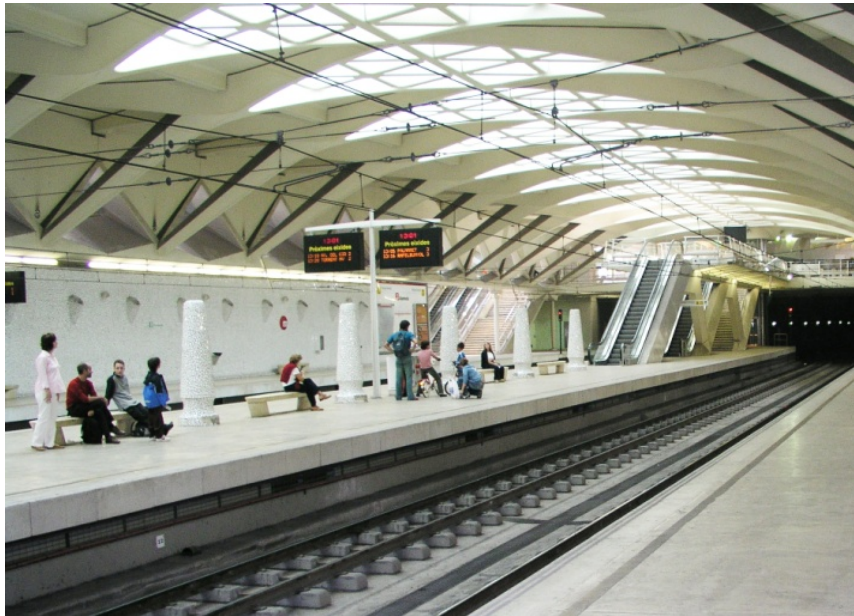
Fig. 6. Skylights in the roof of metro station Alameda , Valencia (Photo: Katarzyna Jasińska).
