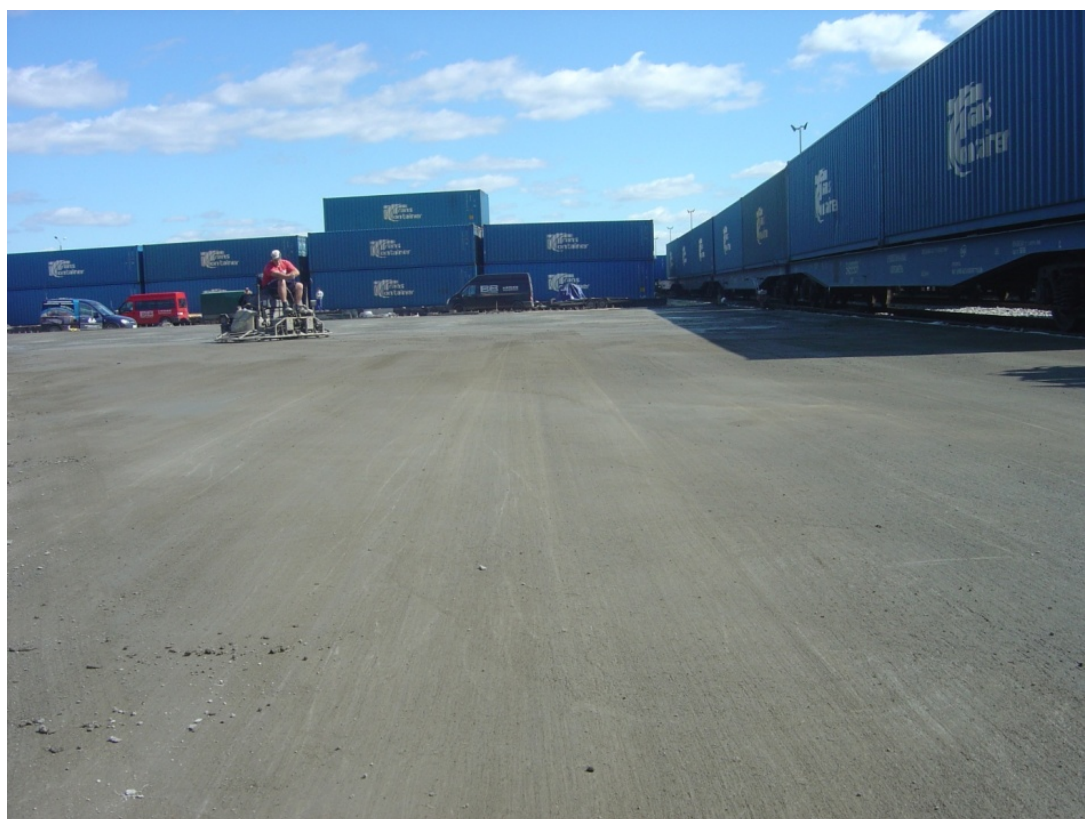
Figure 8. Floating and texturing of concrete pavements
