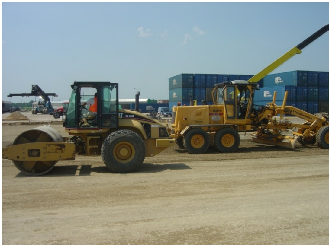
Figure 5. The main foundation is made of mechanically stabilized crushed aggregate
