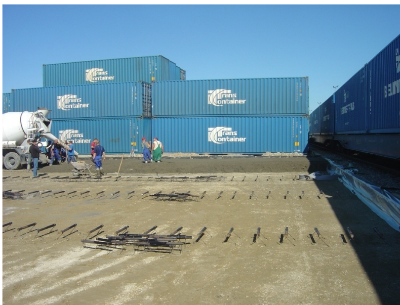
Figure 7. The arrangement of dowels during concreting
