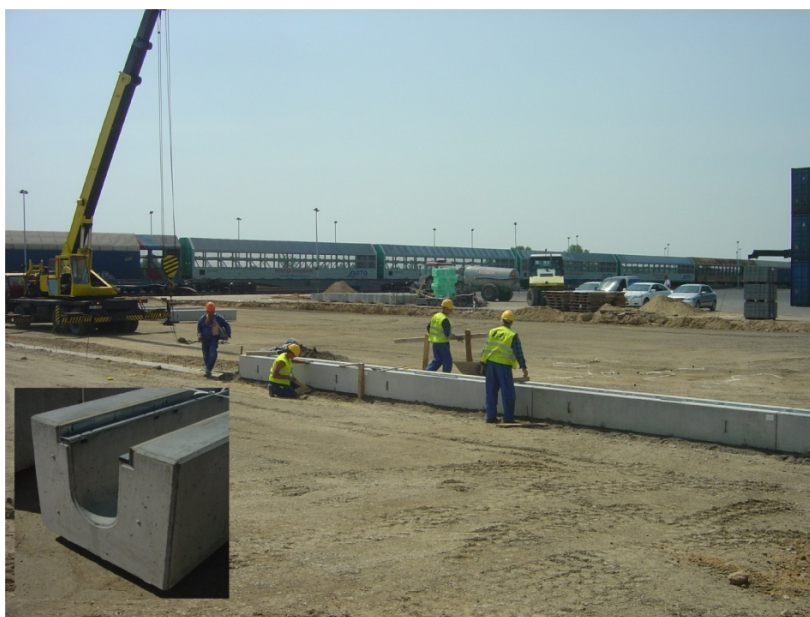
Figure 6. Linear drainage class F 900 made of prefabricated concrete channels
