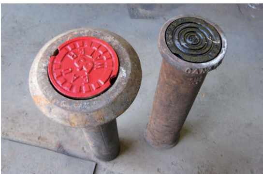
Figure 3. Color codes on covers to indicate whether the water cut-off valve underneath is open or closed.
