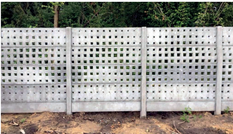
Fig. 5. The “Attractor” fencings realisation at the construction site. Source: [Marcin Giedrowicz]
