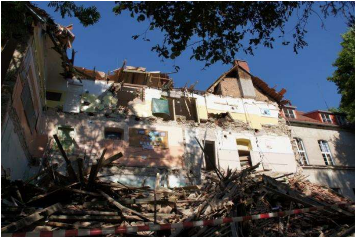
Photo 14. As a result of a gas explosion on the ground floor of the school building (in the food block, in the east wing), the eastern wing was completely destroyed – 31.05.2011 (photo by M. Stachyra)
