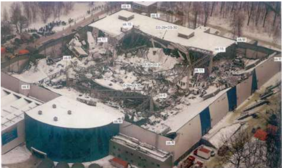
Photo 9. Construction disaster of the exhibition pavilion at the International Fair in Katowice at 1 Bytkowska Street (2006), Source: General Office of Building Control, Warsaw, May 2006.
