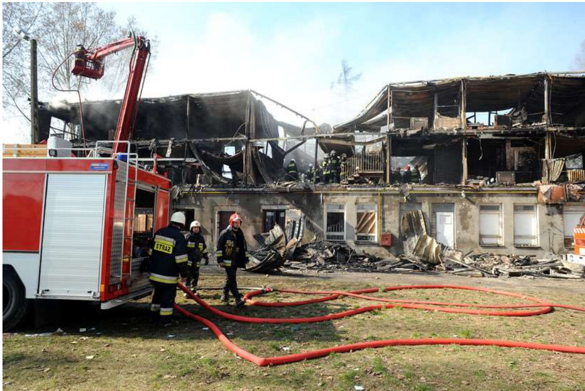
Photo 11. Construction disaster of a three-storey social hotel building in Kamień Pomorski caused by a fire (1995), Source: https://www.rmfm24.pl/fakty/polska/news-pozar-w-kamieniu-pomorskim-urzednicy-skazani-na-wiezienie,nld,1678845
