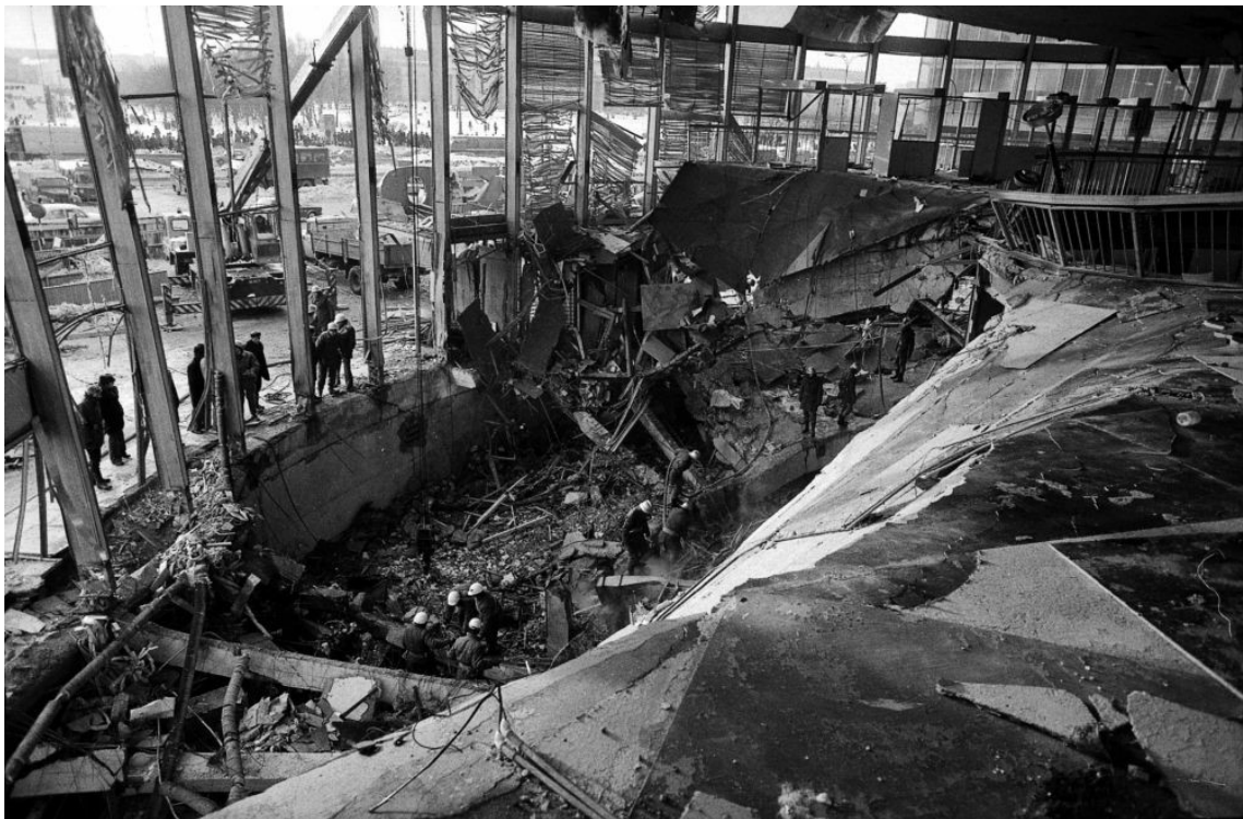
Photo 3. Construction disaster of the PKO Rotunda building in Warsaw (1979) Source: PAP/CAFFoto: M. Kłoś. https://dzieje.pl/sites/default/files/201902/rotunda2.jpg
