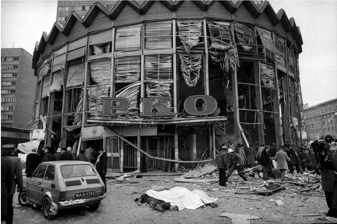
Photo 2. Construction disaster of the PKO Rotunda building in Warsaw (1979) Source: PAP/CAFFoto: A. Urbanek, https://dzieje.pl/sites/default/files/201902/rotunda_0.jpg
