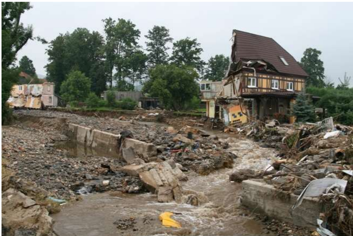
Photo 13. Example of a construction disaster caused by the action of a flood wave resulting from the dam disaster on the Niedów reservoir on the Witka Zgorzelec River,
