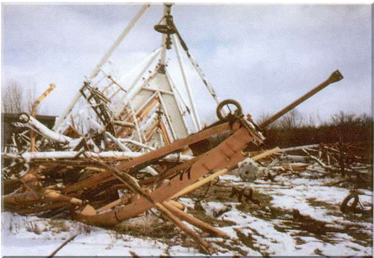
Photo 4. 646 meter mast in Konstaktyńów near Gąbin after the disaster (8.08.1991)
