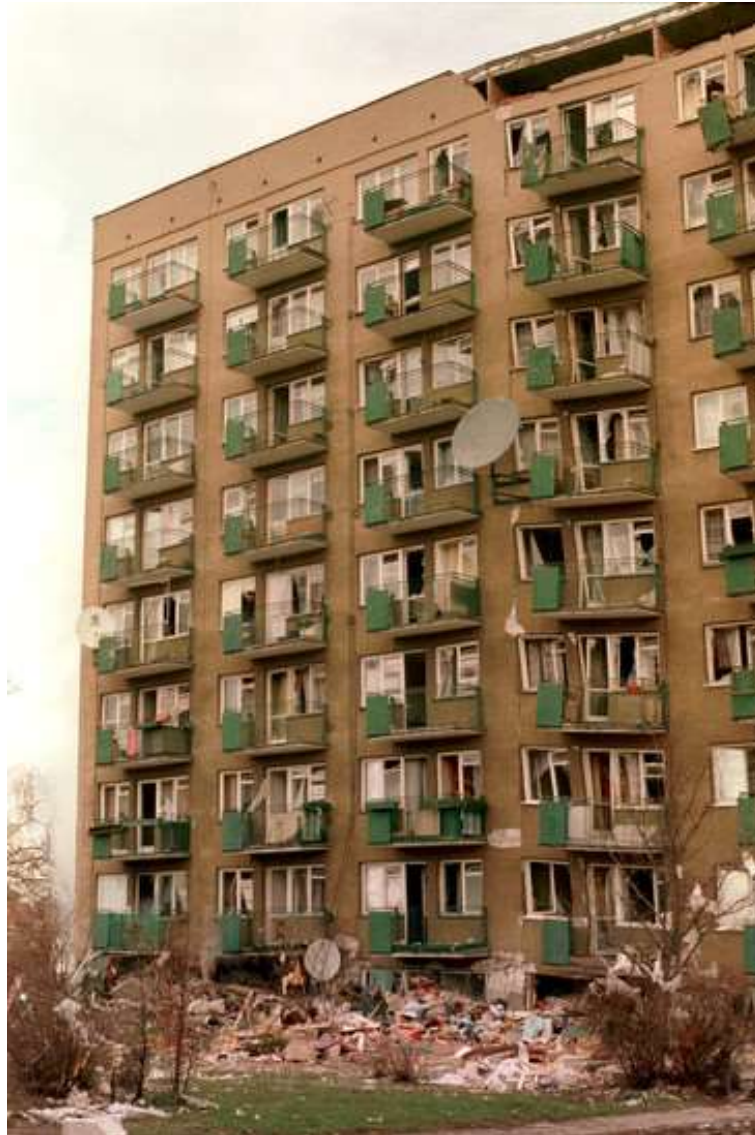
Photo 7. Destroyed multi-family residential building (Gdańsk, 39 Wojska Polskiego Street) as a result of a gas explosion in 1995, Maciej Kosycarz / KFP
