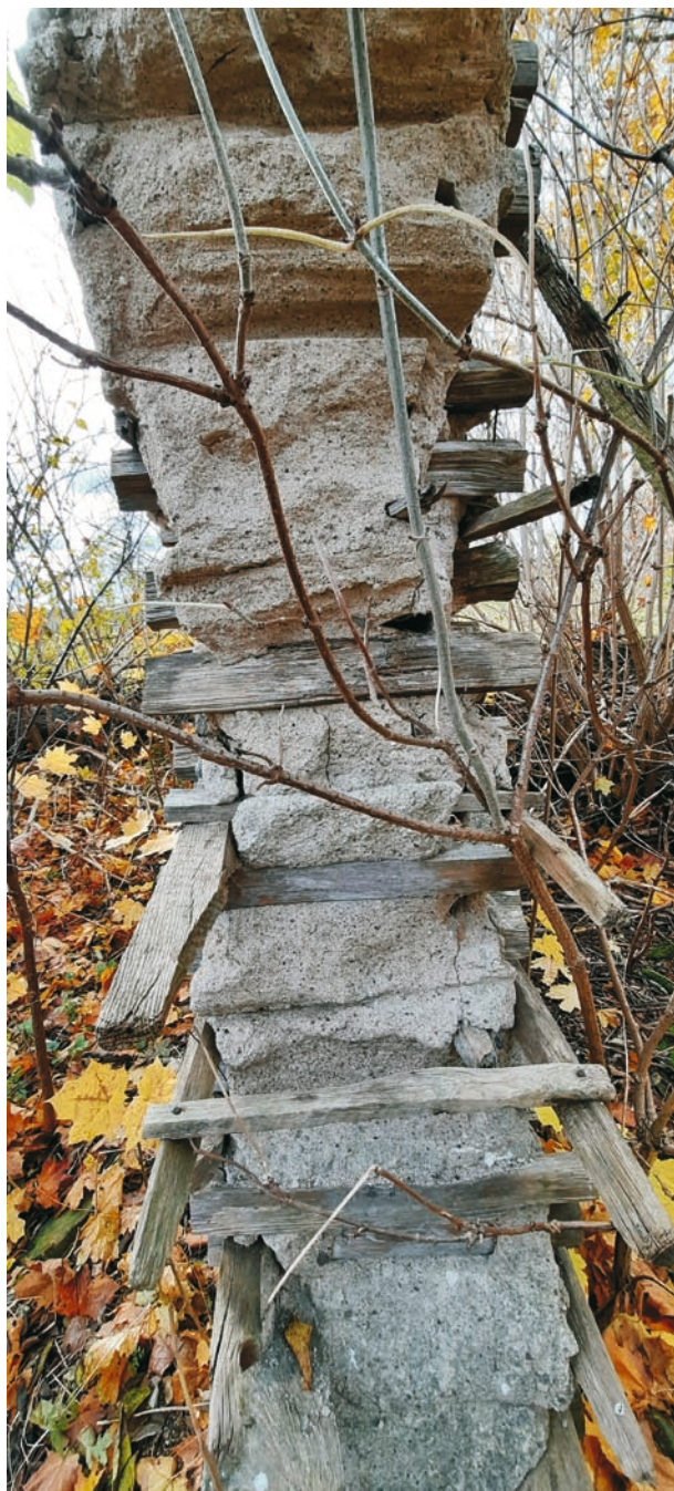
Fig. 8, 9. Cordwood masonry in Rydzewo Kolonia (wall details); photo: Renata Adamska and Katarzyna Karwowska, 2021
