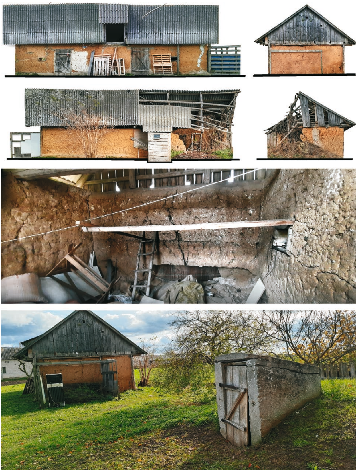
Fig. 15. An old rammed earth barn in Kosilų; photo: Renata Adamska and Katarzyna Karwowska, 2021
