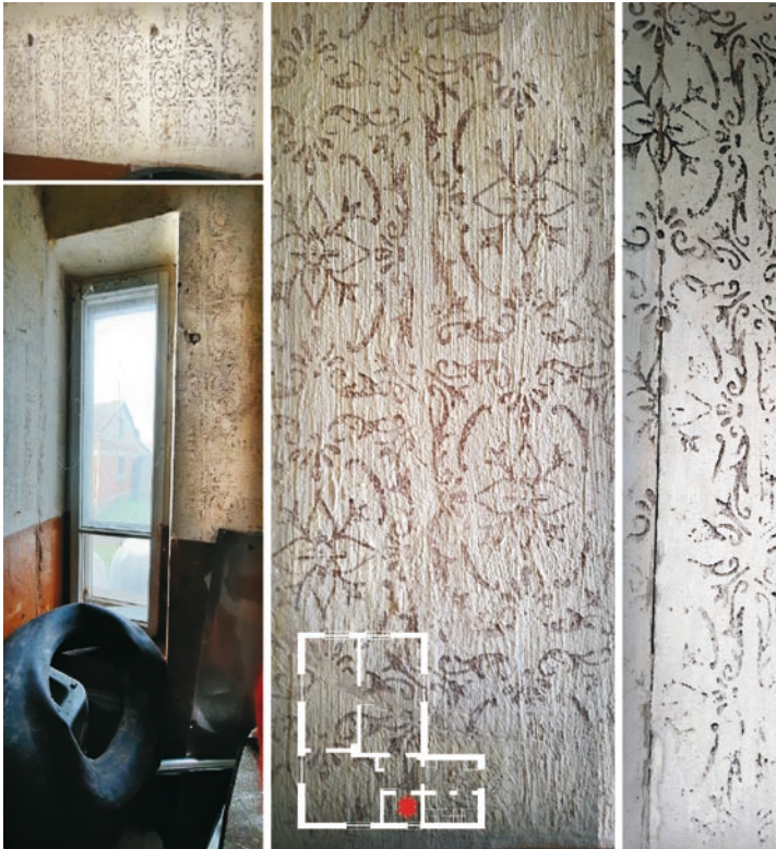
Fig. 18. Stenciled walls in the earthen farmhouse in Konopki Kolonia; source: the authors, 2021
