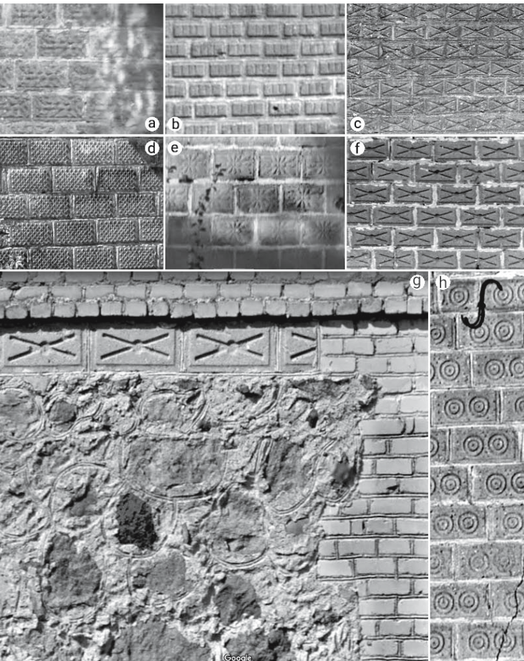
Fig. 22. Hollow brick walls in various villages in the communes of Grajewo and Rajgród: Brzozowa Wólka, Łosewo, Białogrądy, Ciemnoszyje, Flesze, Łosewo, Kolonia Sojczyn Borowy (g, composed with stone and brick masonry), Turczyn (h) - a collection of photos taken in 2012-2022
