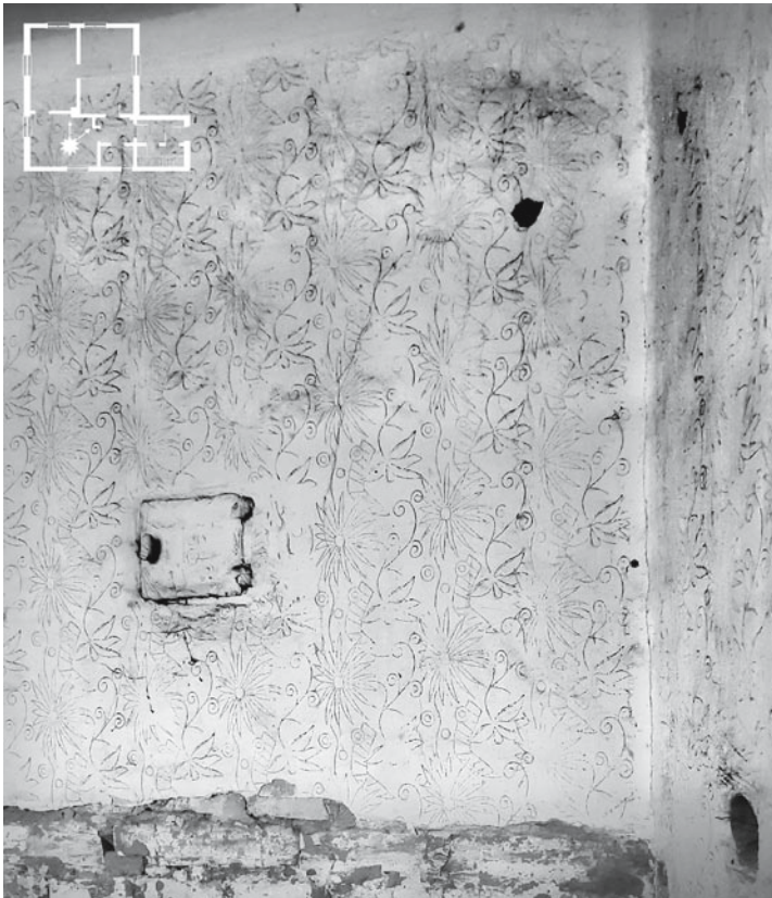
Fig. 19. Stenciled wall in the earthen farmhouse in Konopki Kolonia; source: the authors, 2021
