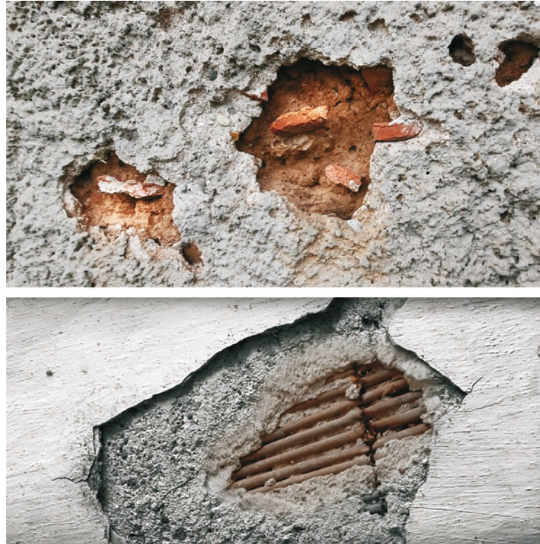
Fig. 20. Wall plaster in the earthen farmhouse in Konopki Kolonia (outer plaster above; inner plaster below); source: the authors, 2021
