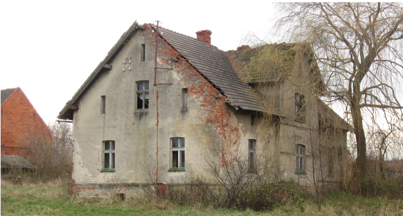
Fig. 1. An abandoned and deteriorating building, 2020
