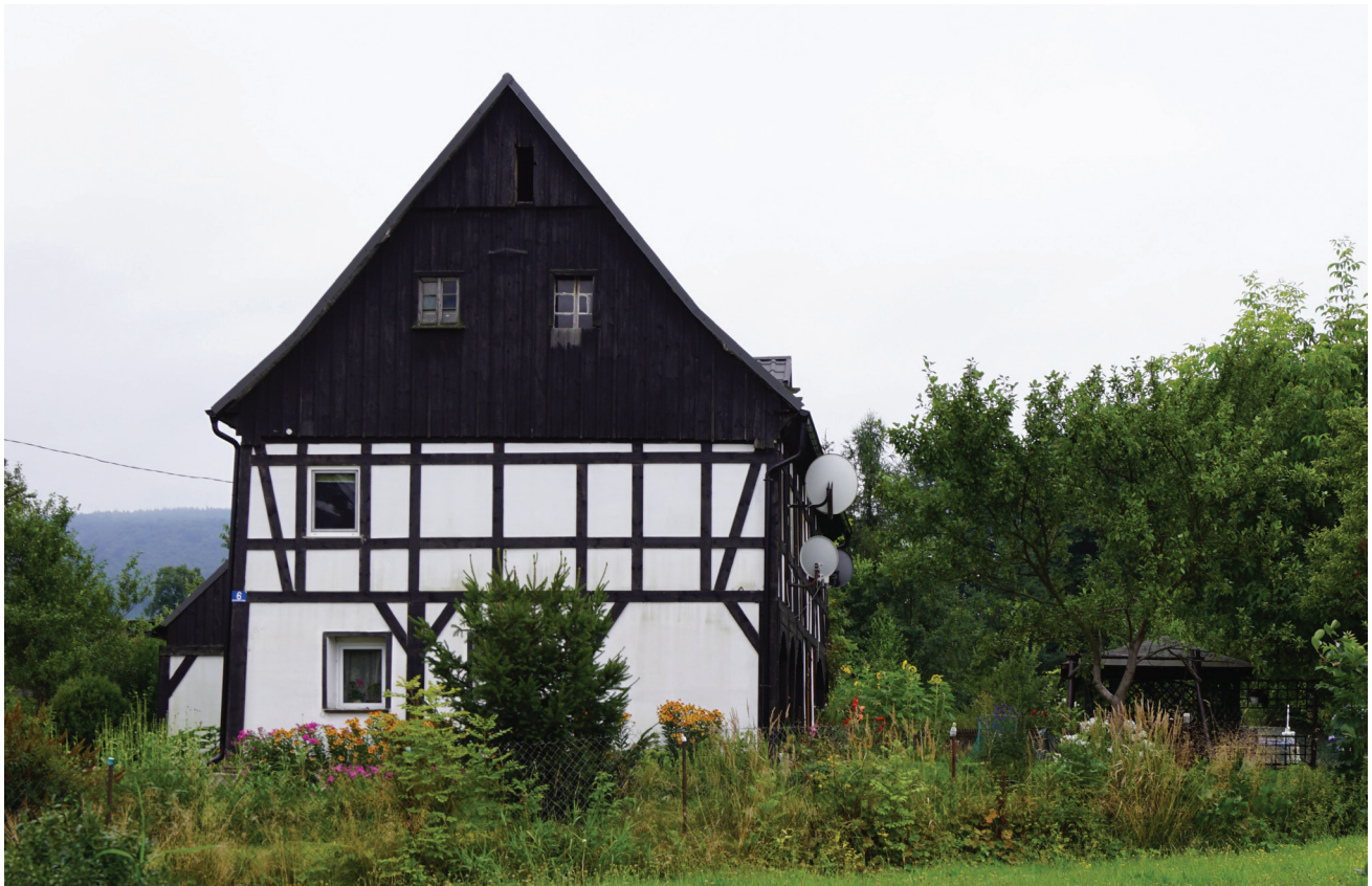
Fig. 2. Building with a half-timbered structure, 2017
