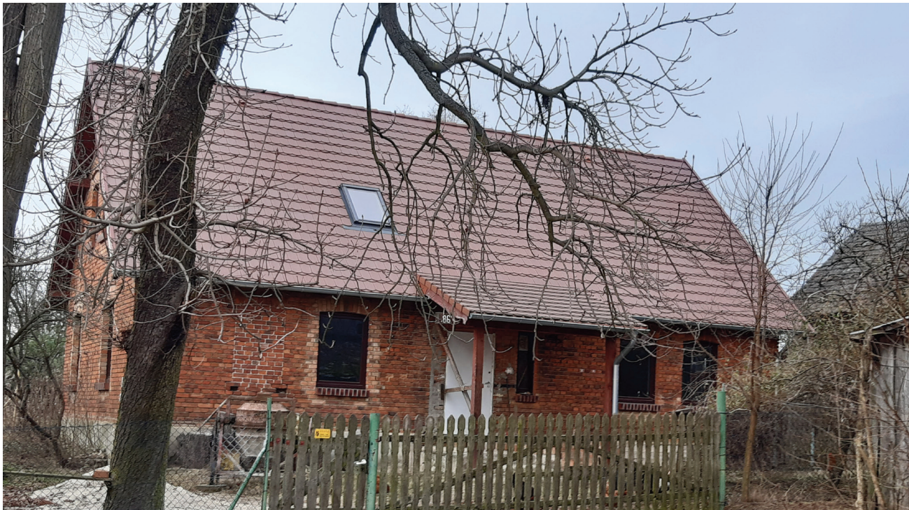
Fig.3. Old brick building under renovation, 2020
