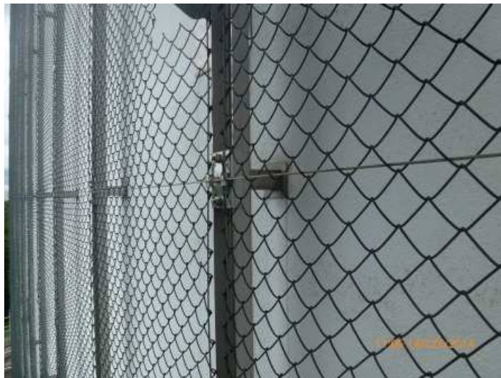
Fig. 6. Construction for green wall - Philharmonic Hall in Białystok
