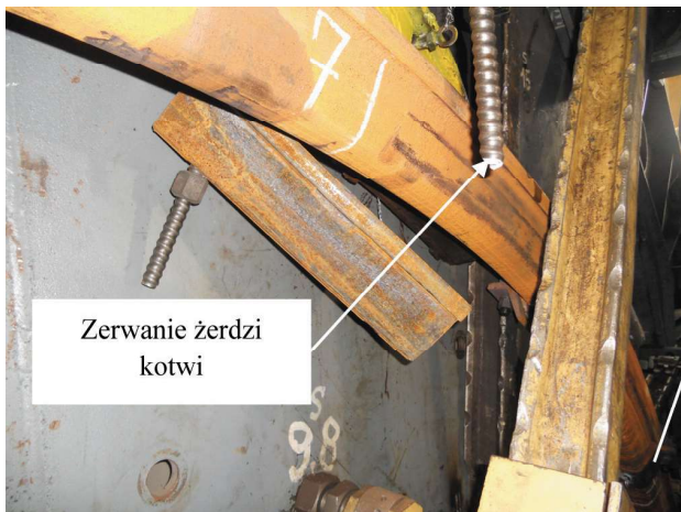
Fig. 6. Dependence charts of the frame loading force F and the forces in the roof bolts as a function of time t
