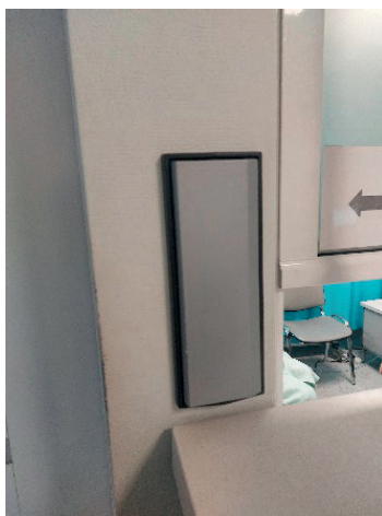
Figure 11. The mechanism of opening a door with a button using an electromagnetic lock
