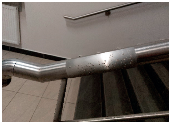
Figure 10. Information plates in Braille placed on the balustrades
