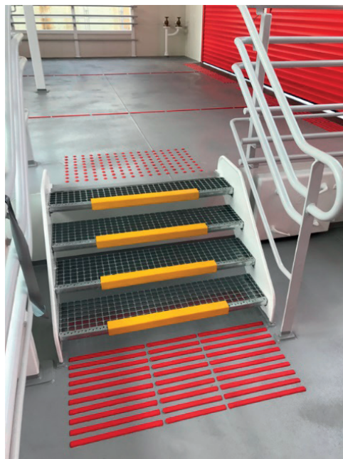
Figure 15. An example of marking stairs inside the building for the visually impaired
