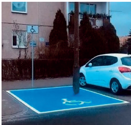
Figure 8. An example of an inappropriately located parking space for people with disabilities
