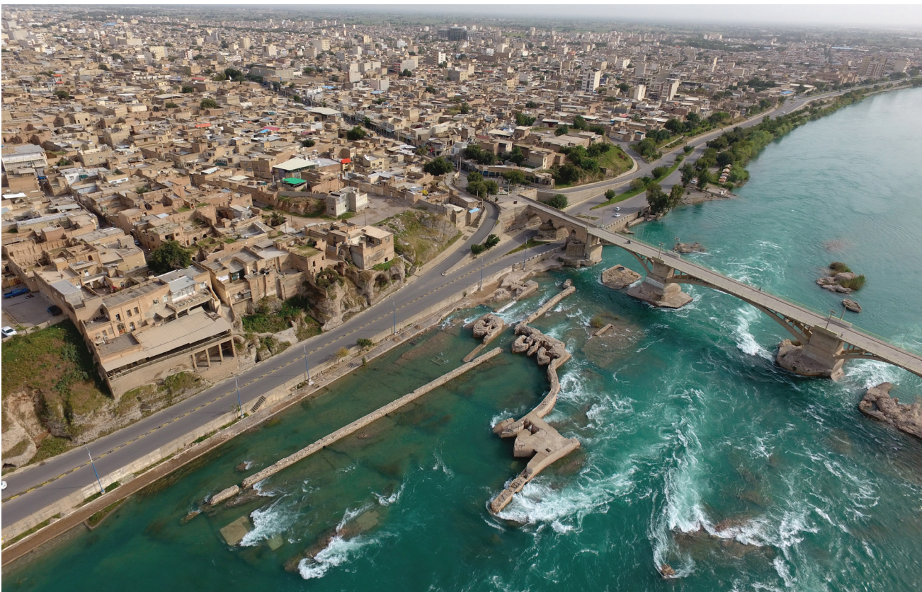
Fig. 3. Watermills of Dezful after the flood – 2016; source: Ramin Karamzadeh
