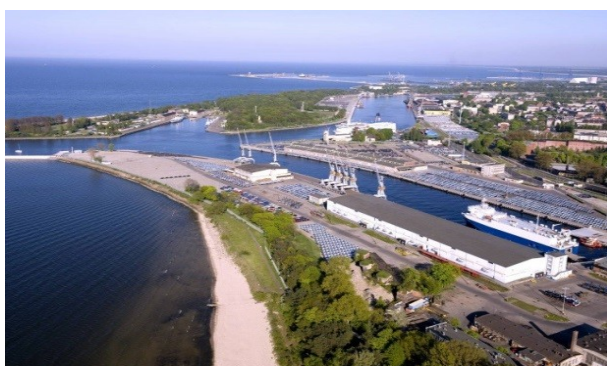
Fig. 3. The WOC II Quay in the port of Gdańsk [15]
