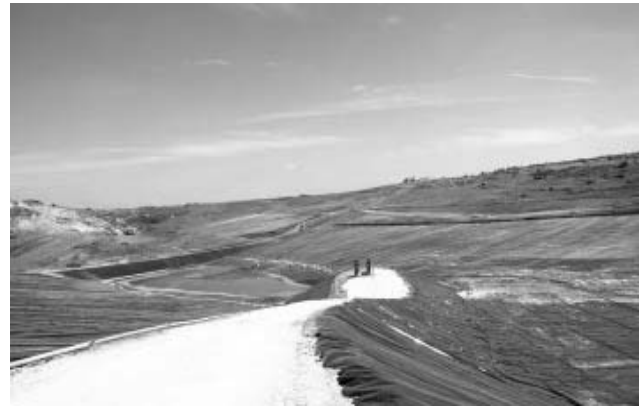
Fig. 2. Landfill with an impervious sheet cover
