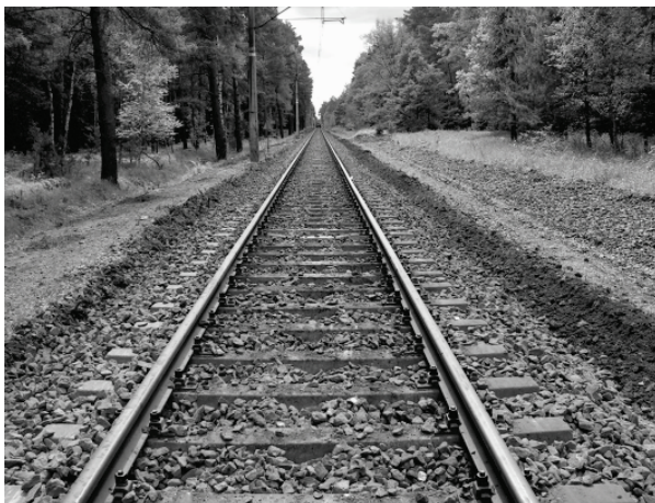
Fig. 8. View of the section of track No. 1 on line No.279 Luban – Wegliniec after the modernization. Source: M. Winiarski [3].
