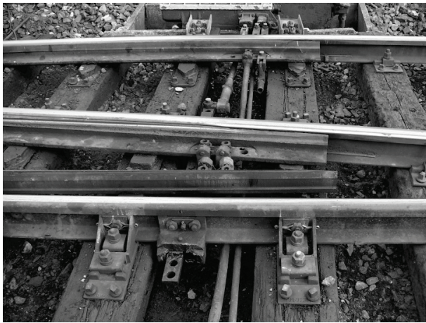
Fig. 2. A fragment of the double crossover turnout (like 60E1) with a chipped half-turn switch and notable side consumption of the needle [3].
