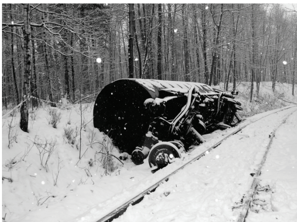
Fig. 6. wagon derailment of a freight train, which consequence was a serious damage to the track (destruction of the geometric plan and longitudinal profile).
