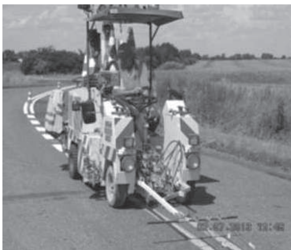
Fig. 1. Markings are mechanically applied on the road [author's photograph].
