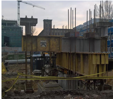
Fig. 3. View of loading structure of the barette B81 (author's photo)
