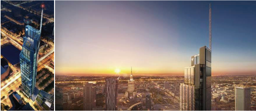
Fig. 1. View of the designed building and its 80-metre mast – a "bird's eye view"
