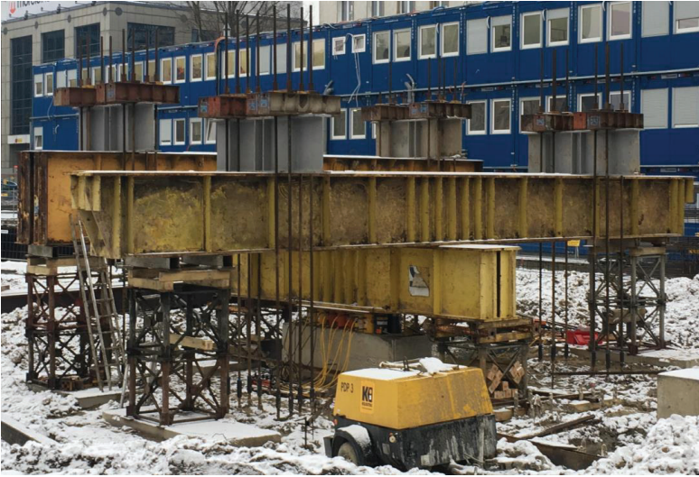
Fig. 2. View of loading structure of the barette B82 (author's photo)
