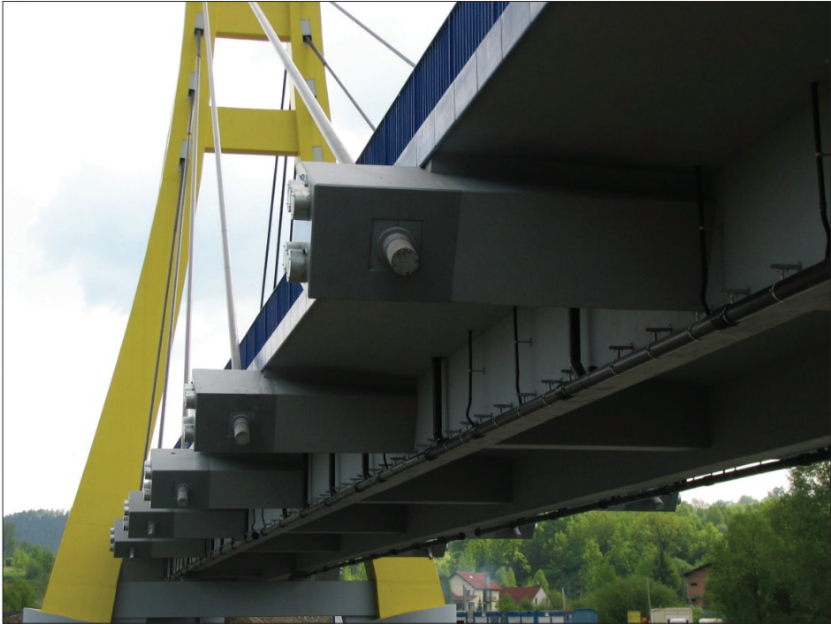
Fig. 1. The span of the bridge measured with a radar system (radar unit located next to the pylon)
