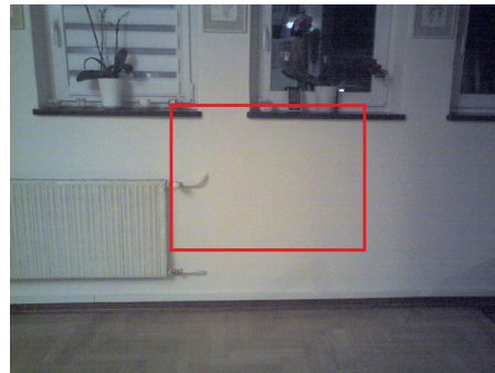
Fig. 5. Photo of the wall No. 2 – 8/01/2018
