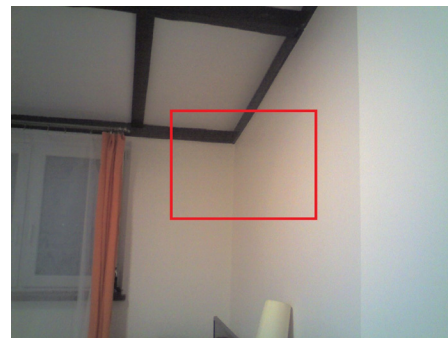
Fig. 7. Photo of the wall No. 3 – 8/01/2018
