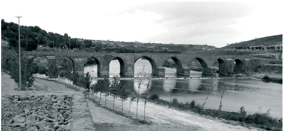
Fig. 3. Upstream elevation of Bridge, [6]
