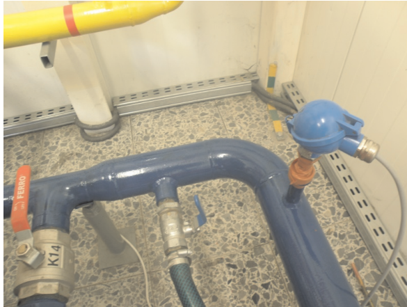
Fig. 3. Transducer of final temperature of a heating medium Phot.: Authors
