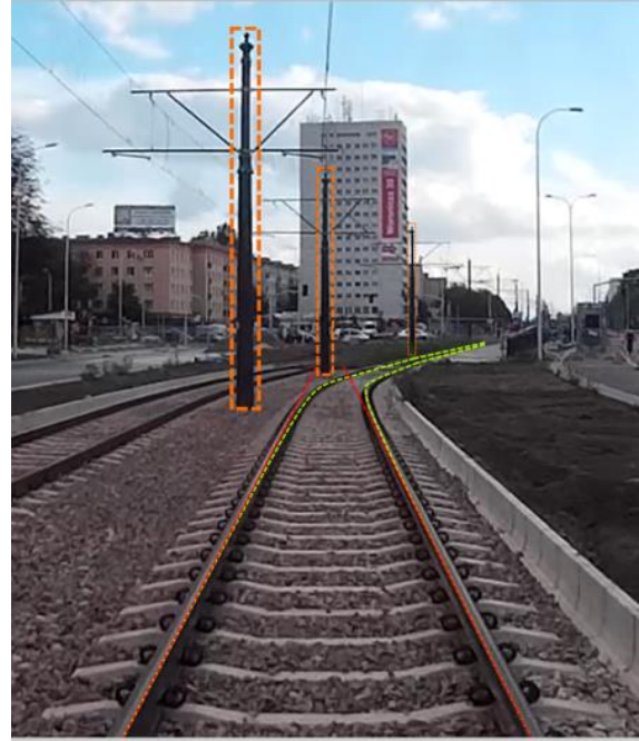
Fig. 1. Trajectory of tramway movement a) crossing of the tracks with road, b) catenary pylons close to track curve
