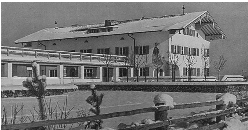
Fig. 10. Airport in Ainring; source [27]
