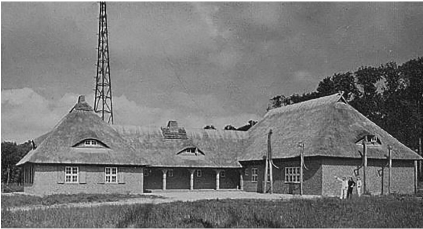
Fig. 11. Weather service radio station on Sylt; source [27]
