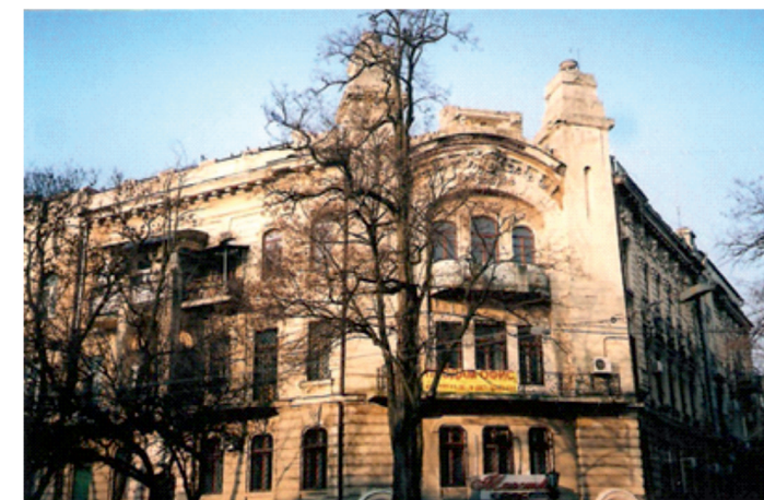
ill. 4. The house at 2 Marazliivska Street in Odessa. Photo: Yu. Ivashko
