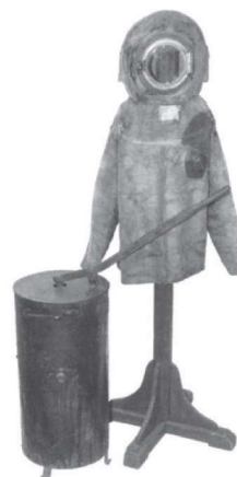
Rys. 2. Aparat oddechowy ROYGUAYROLA - 1862r. Fig. 2. ROYGUAYROL breathing apparatus - year 1862
