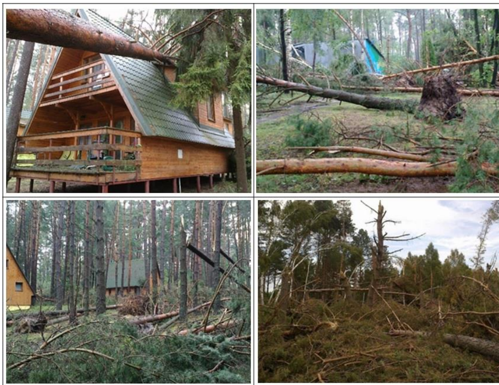
Phot. 2. Damage of tree stand and an infrastructure of ATC Czernica [photo C. Dyrzcz]
