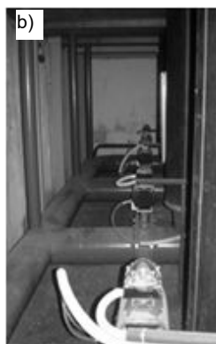
Phot. 1. Contact polystyrene foam filters of Teteryv River water treatment: a) top view; b) flushing valve with pneumatic actuator (photo: S. Martynov)
