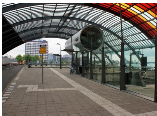
Fig. 2. Bus station at the railway station Amsterdam Centraal. Source: author
