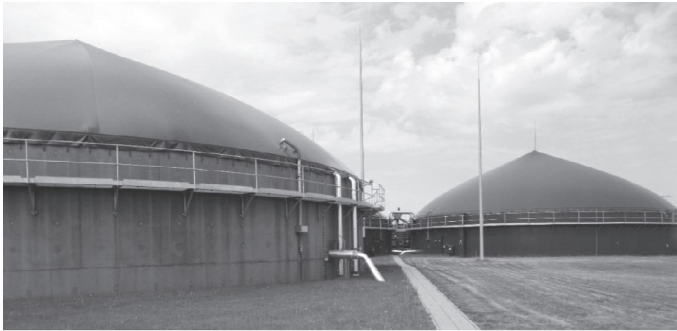
Fig. 2. The storage tank and fermentation chamber located in the Ryboly Biogas Plant
