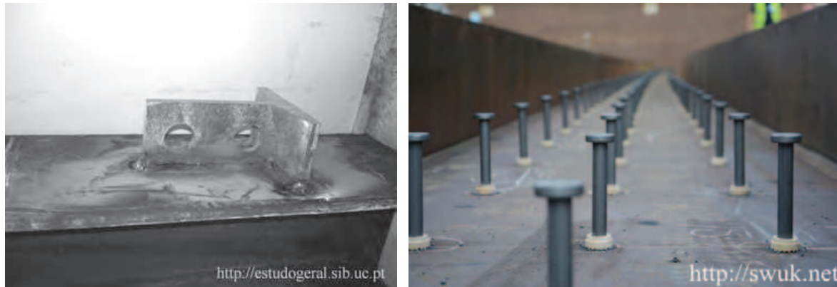
Fig. 1. Examples of discrete connectors
