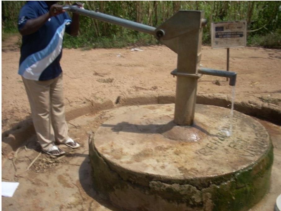
Plate IV: A community hand-dug well mounted with hand pump in the study area. This well retains sufficient water all-year round
