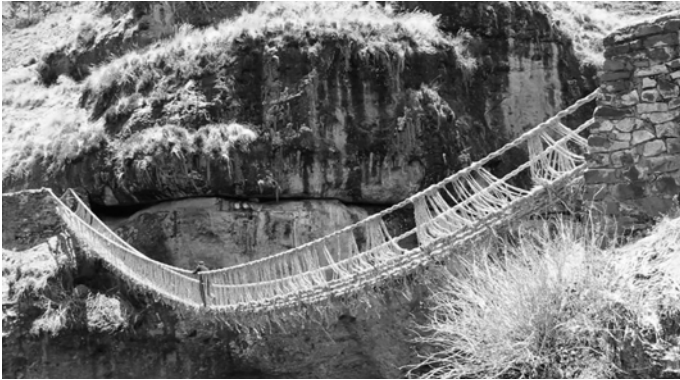
Fig. 2. Keshwa Chaca – suspension bridge in the Andes, rebuilt by the local community with the use of techniques applied in the past. Source: [11]
