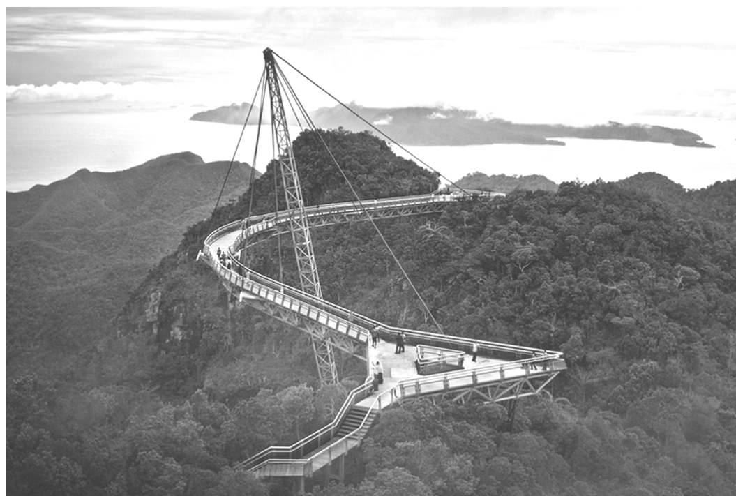
Fig. 11. Cable-stayed structure of Langkawi Sky Bridge. Source: [29]
