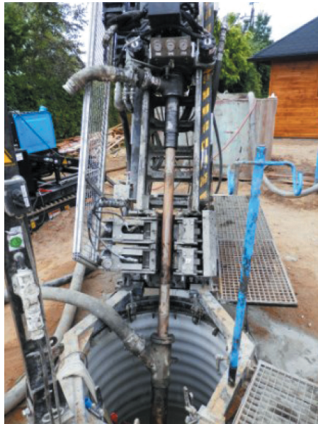
Fig. 8. Drilling without casing pipes with a preventer [2]
