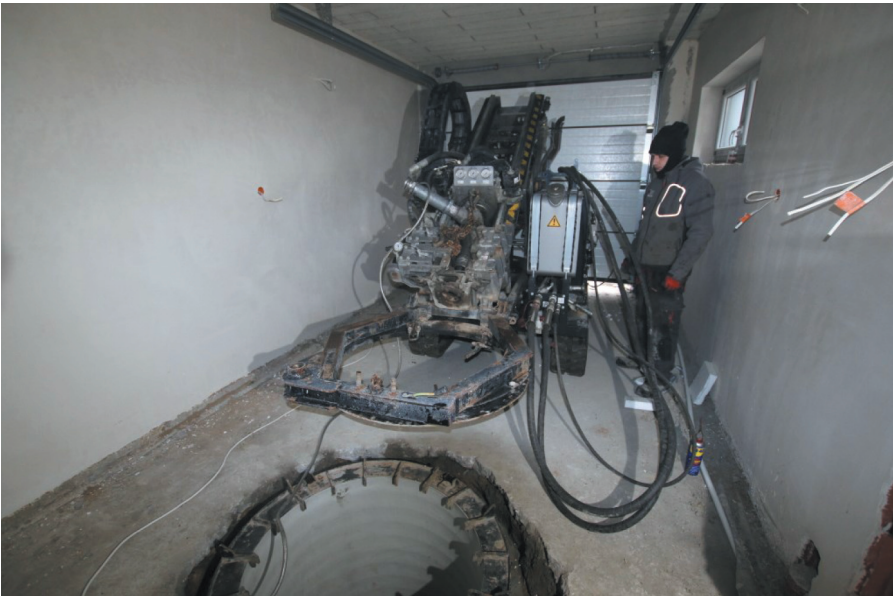
Fig. 15. Preparation prior to drilling in a garage (OPTIMA POLSKA 2015)
