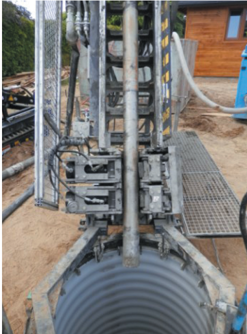
Fig. 7. Casing pipes with a drilling crown [2]
