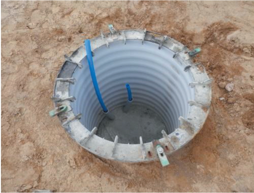
Fig. 1. A drilling chamber with a ring mounted onto it. Two connecting tubes are visible inside [2]
