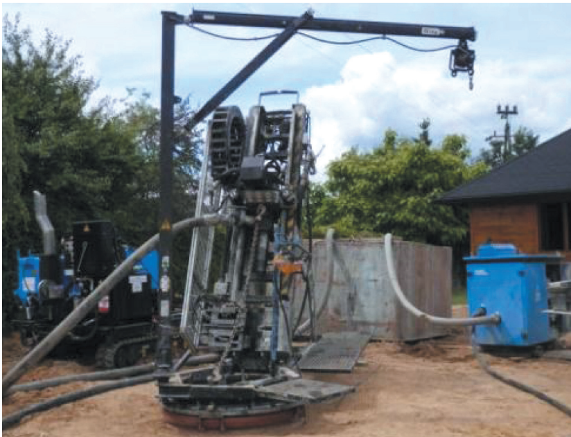
Fig. 6. Equipment ready for drilling [2]
