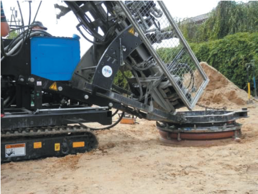
Fig. 3. Setting the drill rig onto the chamber [2]
