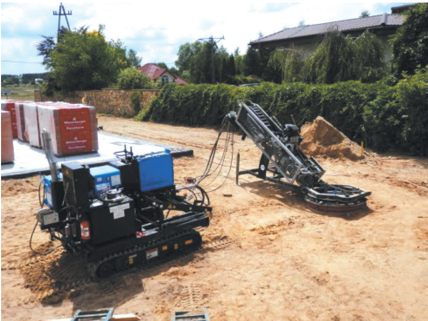
Fig. 4. The driving unit and the drill rig [2]
