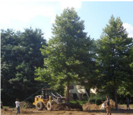
Fig. 19. Tree relocated with its entire, pre-cleaned root system. Source: Taking
