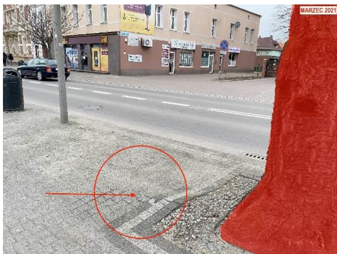
Fig. 13. Tree at Konstytucji 3 Maja in Goleniów after the laying of concrete pavers around its trunk, same location, photo made 3.5 years later in March 2021. Source: author.
