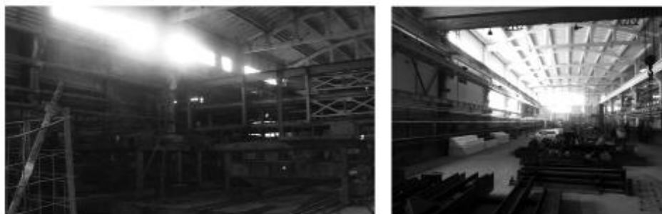
Figure 5. (A) General view of molding span No. 1 before modernization; B) General view of the molding span N \underline{0} 1 after modernization
