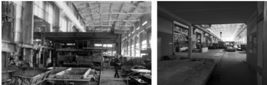
Figure 21. A) General view of molding span No. 4 before modernization; B) General view of the molding span No.4 after modernization
