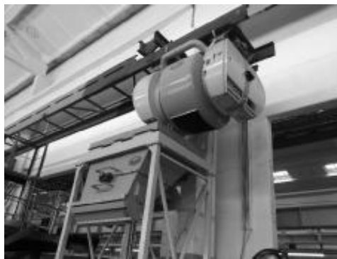
Figure 25. Post reception of concrete mix from Kubel of address giving
