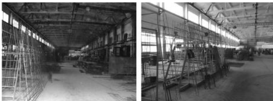
Figure 2. a) General view of the reinforcement shop before modernization; b) General view of the reinforcement shop after modernization
