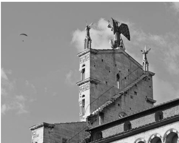
Fig. 7. View at the back of façade.
