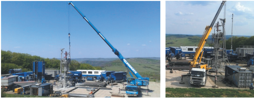
Fig. 9. Snubbing unit working on the field
